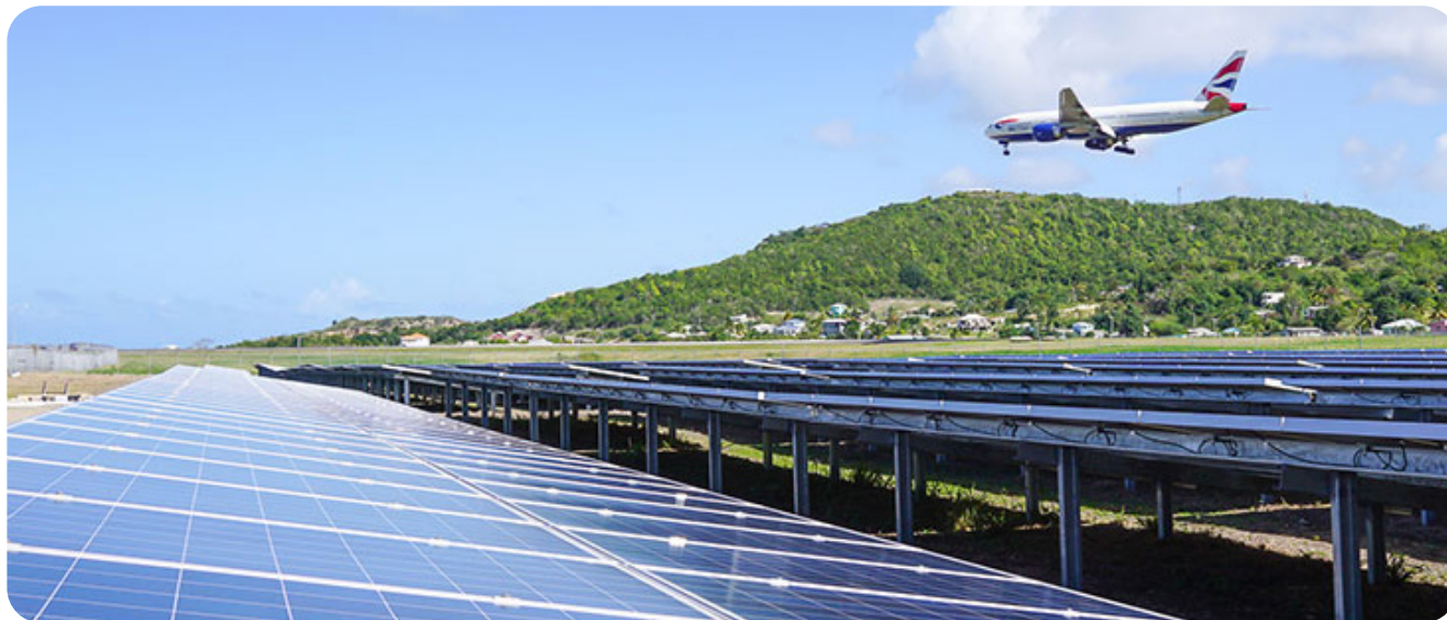
RLB Airport Solar Farm
